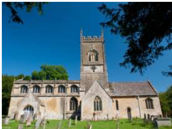
St Michael and All Angels in Withington, Gloucestershire, claims to be the country's first zero-carbon church with solar panels mounted on the hidden section of the flat roof
